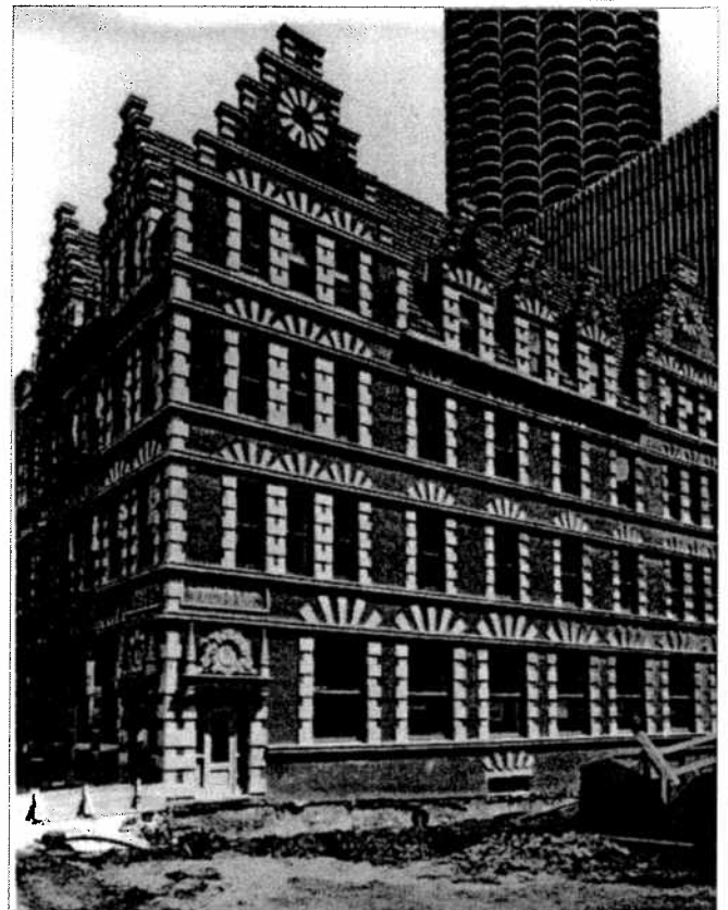
1963: The Dearborn Street facade as it appeared when the street-level was being raised. The new street viaduct obscures the basement level window visible in this photo.
